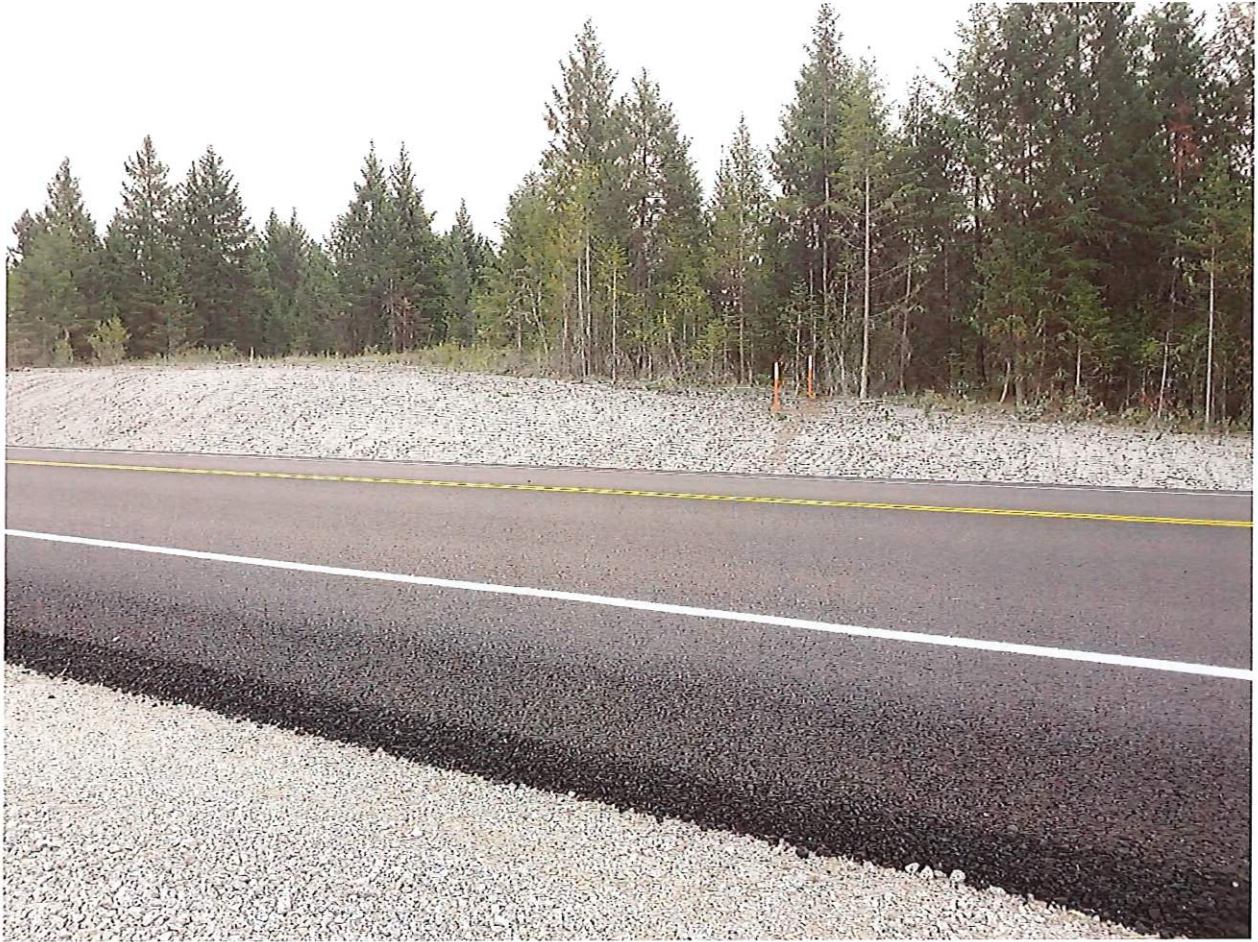
Facing East (Green Stakes)
