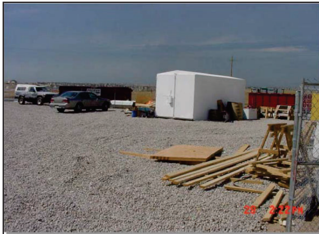
Figure 98. Construction staging area (Colorado UDFCD 2010).
