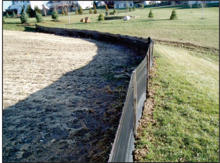
Figure 157. Silt fence (York County Conservation District 2009).
