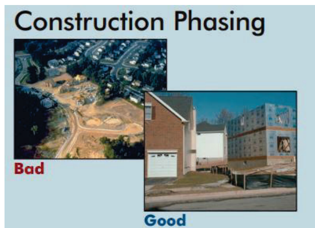
Figure 97. Construction phasing reduces the amount of time soil is exposed (EPA 2003).
