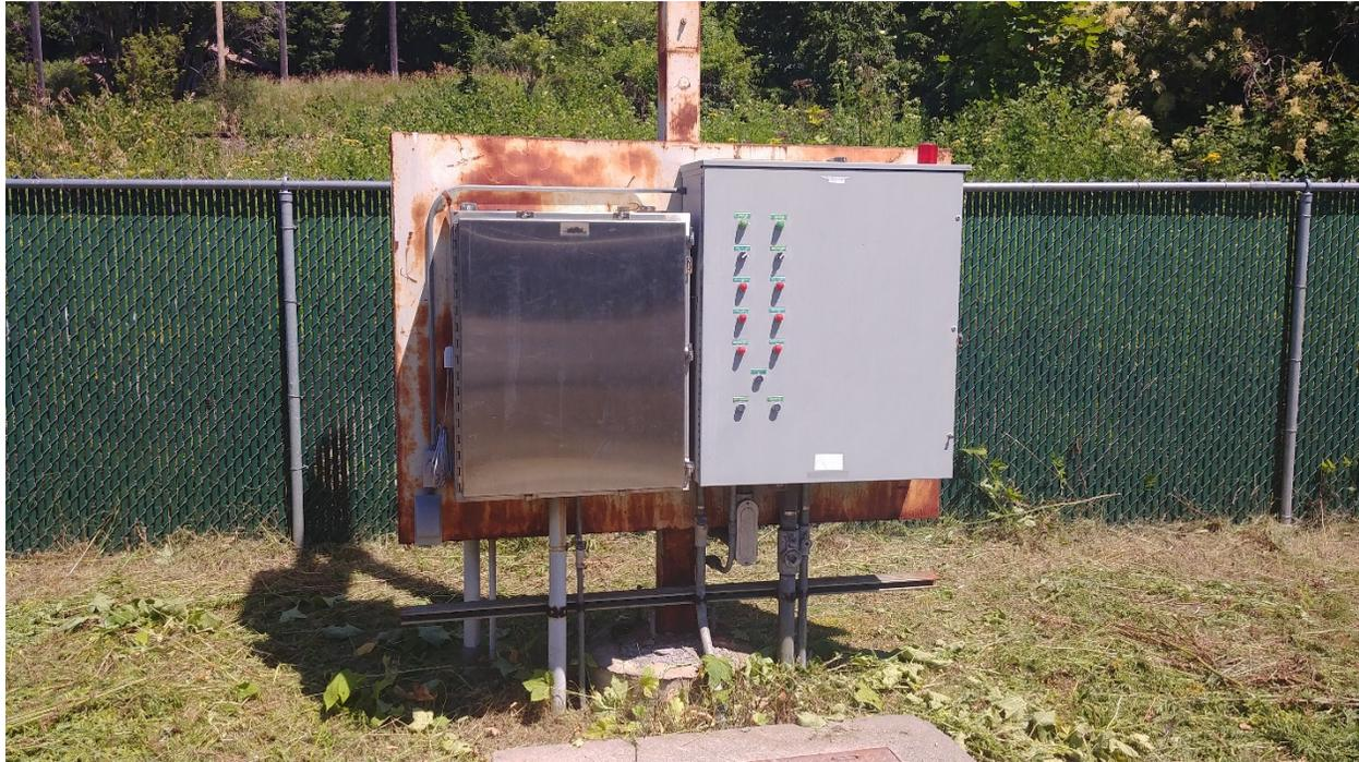
**Photo 2 - Lift Station Control Panels**
