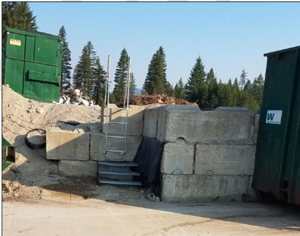
**Exhibit 3-7. Failing Eco-Block Retaining Wall (Dickensheet)**
