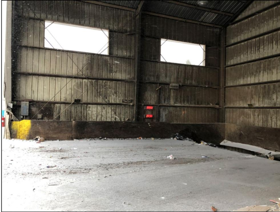
**Exhibit 3-3. Waste Transfer Building Interior Showing Floor and Push Walls (Colburn)**
